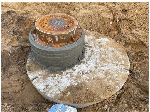
Photo #9: Manhole with adjusting rings, frame, and cover. - Nov 14, 2023, 8:43 AM
