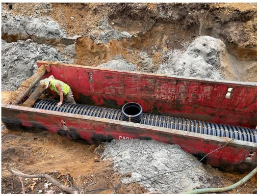
Photo #4: Gravity pipe with 18" riser pipe portion on top - Oct 24, 2023, 2:07 PM
