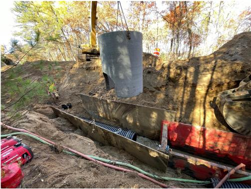
Photo #2: Installing manhole - Oct 23, 2023, 1:19 PM
